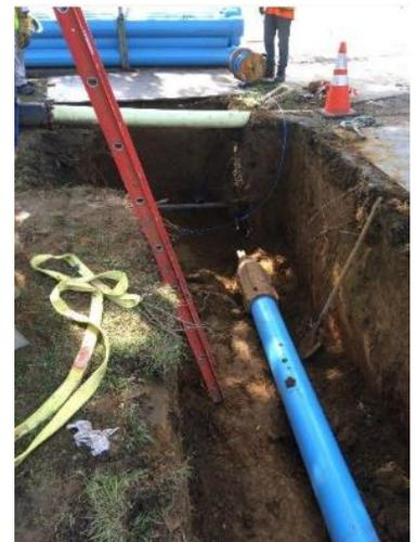
**Heather Hills:** After completion of a hydraulic analysis, 0.4 miles of piping has been identified to be replaced along Hillman Place and a large section of Holiday Lane. This project includes some 'open cut' work (pipe expose by digging), and some pipe bursting as described above.
