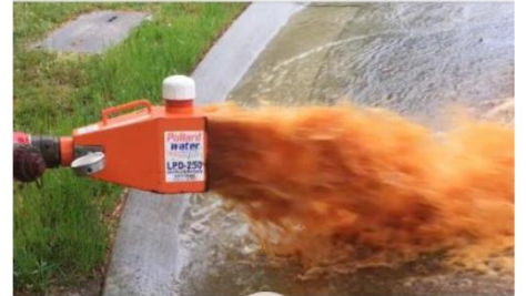
Hydrant Flushing, City of Bowie
